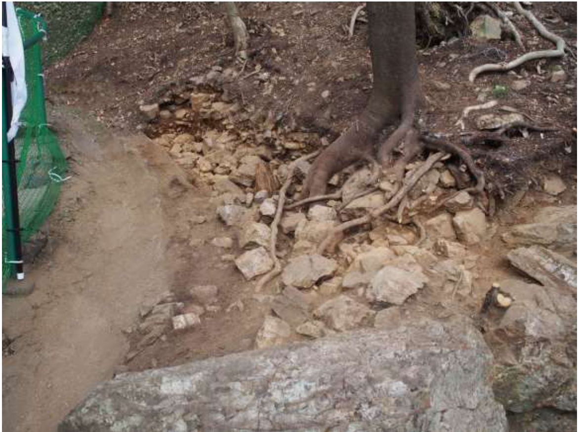
1区石垣 裏込め
