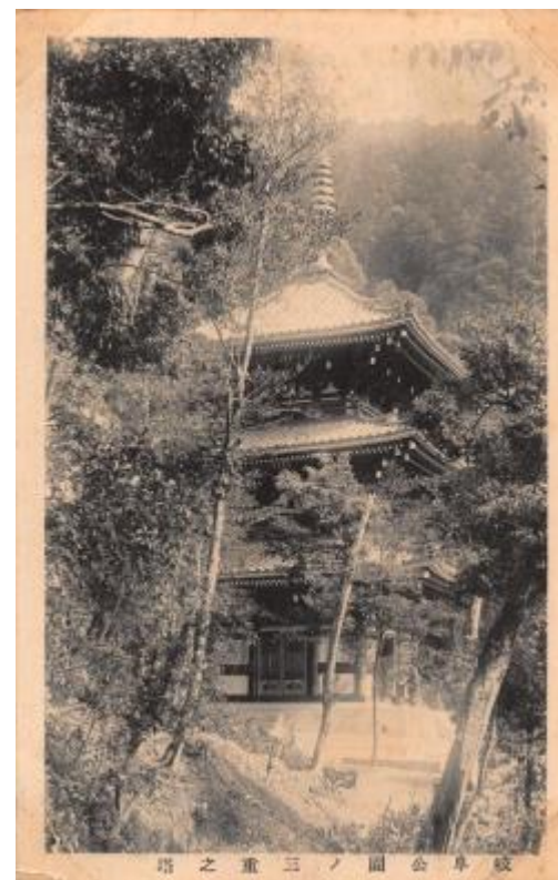
A photograph of the three-storied pagoda taken at the time of completion
