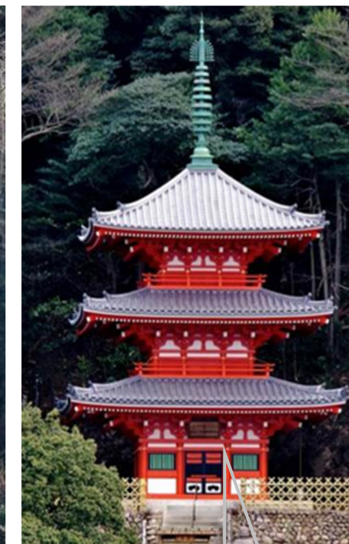
Pagoda after restoration was finished (2017)
